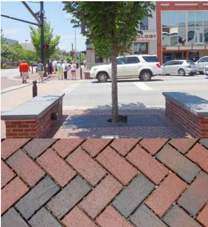
Permeable pavers and suspended pavement support this tree’s health by allowing more water to reach the tree’s roots, providing additional structural support as the tree grows, while reducing runoff.
