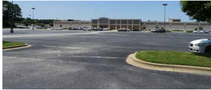
Excess impervious areas cause hot temperatures and runoff. Some older paved areas predate regulations requiring stormwater management.
