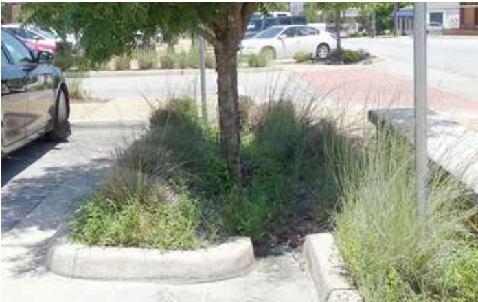
This municipal parking lot next to city hall has a bioswale – a recessed bed planted with a tree to capture and clean stormwater before it reaches the city drainage system.
