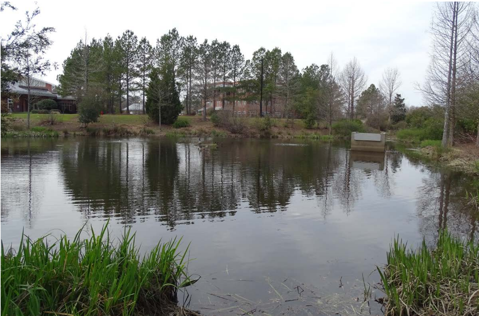
Vegetated stormwater pond helps detain and clean runoff.
