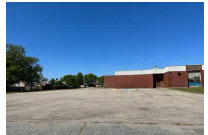
Excess impervious areas cause hot temperatures and runoff. This parking lot can be retrofitted to add more trees.
