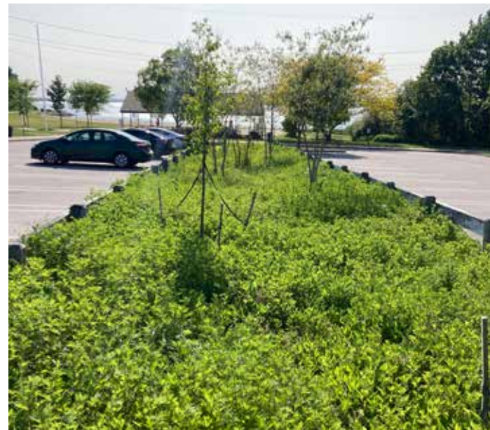
These recessed tree islands in the Bristol Town Beach parking lot are a good example of integrating trees into Low Impact Design (LID) which slows, filters, and reduces stormwater entering the bay.
