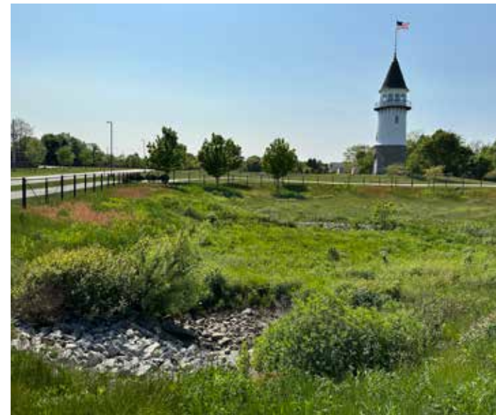
Stormwater basins can be planted with trees where maintenance access is not prohibited to provide additional stormwater capture.
