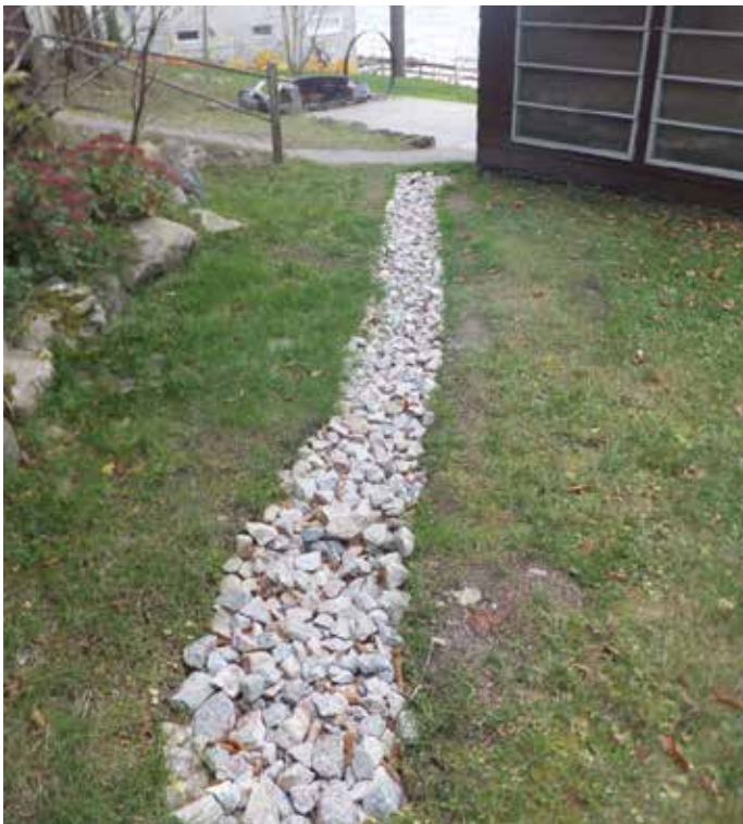
Infiltration trenches are a low-cost, low-tech way of reducing urban stormwater runoff on private property. This type of practice is compatible with tree plantings for added stormwater mitigation value.
