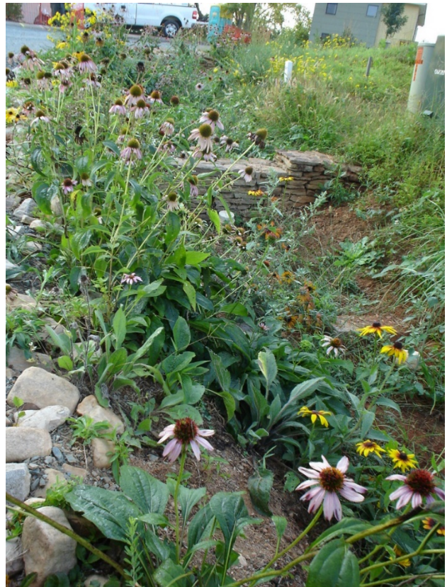
Bioswale at Riverbluff Circle slows and cleans runoff
