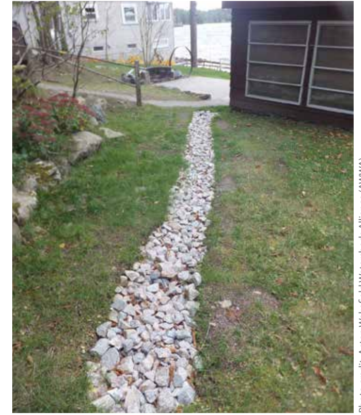
Infiltration trenches are a low-cost, low-tech way of reducing urban stormwater runoff on private property. This type of practice is compatible with tree plantings for added stormwater mitigation value.
