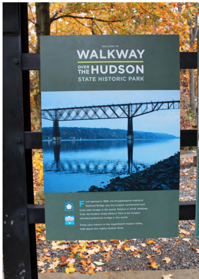
Hudson walkway sign.
