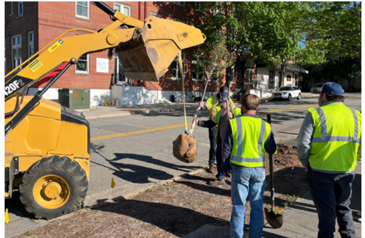
Field crew members install trees in downtown tree pit.
