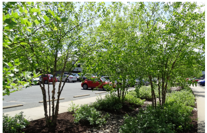
Parking lot with bioretention basin in continuous linear parking strip between parking rows.
