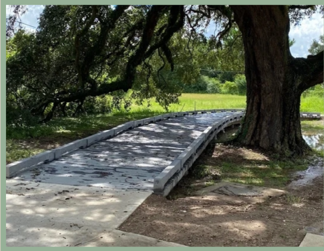
Bridging the sidewalk with a wood or metal boardwalk
