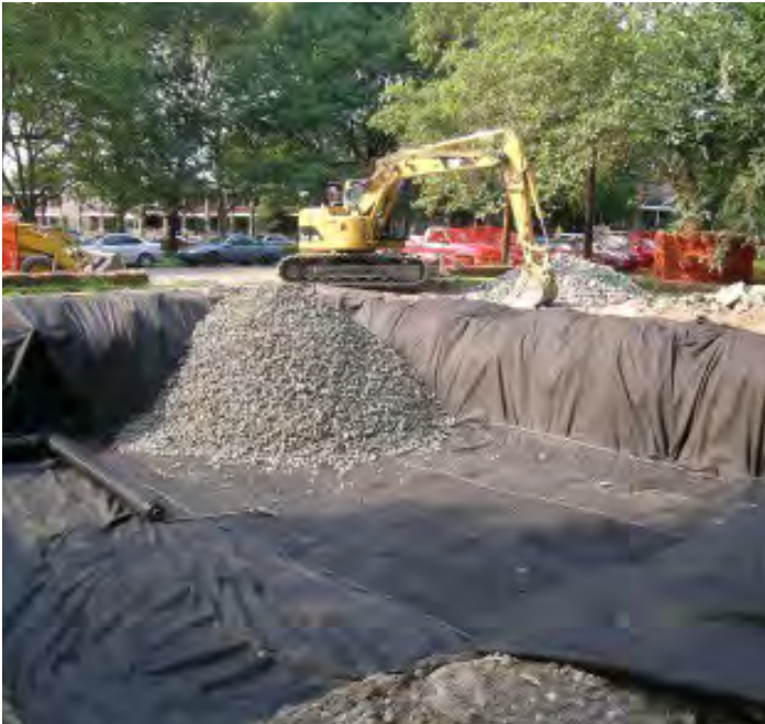
Construction of the basketball court at Clark Park shows the installation of material to allow water to percolate through with a liner to trap finer materials.
