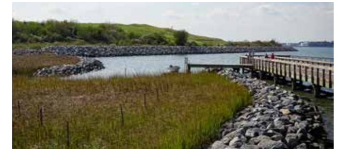
This shoreline restoration project used a combination of living shorelines and rocks to ensure the habitat is protected from strong wave actions.
