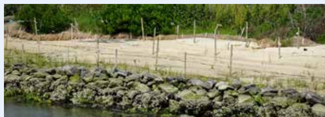
Shoreline restoration project underway.
