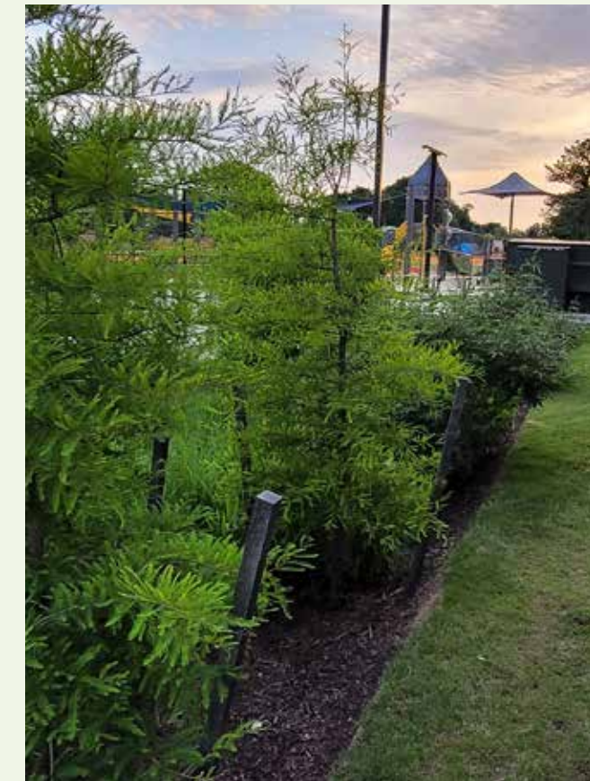
Bioswales were installed to capture roof runoff at the new Mary Jackson neighborhood center.
