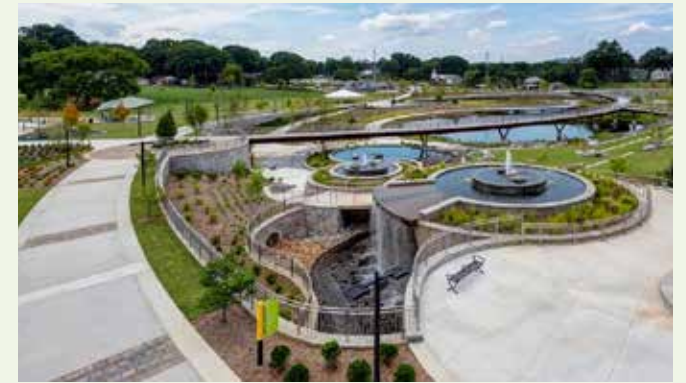
Rodney Cook Sr. Park in Atlanta reduces flooding by capturing and storing up to 10 million gallons of stormwater while simultaneously creating a vibrant community destination.
