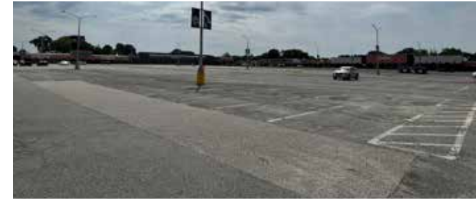
Excess impervious areas cause hotter temperatures and increased runoff. This parking lot at Cavalier Square could be retrofitted to add more trees, bioswales, and pervious surfaces that allow water to seep into the ground.
