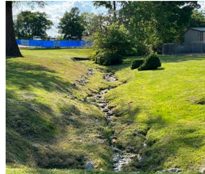
Adding trees and other riparian species along this channel along Elm Street would slow water during rain events, allowing for more infiltration into the soil.
