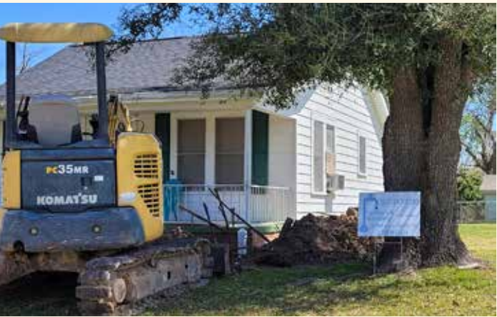
This tree is not adequately protected from ongoing construction. Heavy machinery can compact the soil, damage roots and lead to decline in tree health or mortality.
