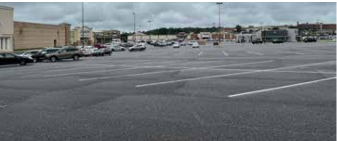
Excess impervious areas cause hotter temperatures and increased runoff. This parking lot could be retrofitted to add more trees, bioswales, and pervious surfaces that allow water to seep into the ground.
