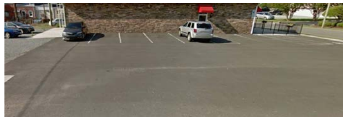
Excess impervious areas cause hot temperatures and runoff. Some older paved areas predate regulations requiring stormwater management. This parking lot can be retrofitted to add more trees
