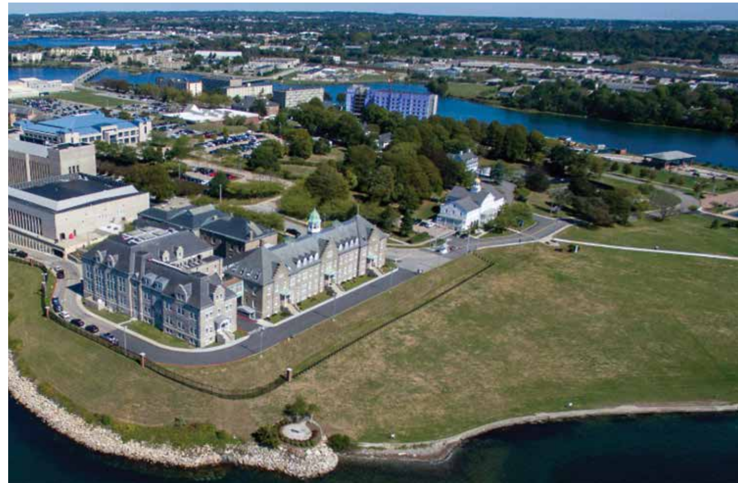
The U.S. Navy owns much of Newport’s land, where tree canopy covers less than 10% and impervious surfaces dominate.
