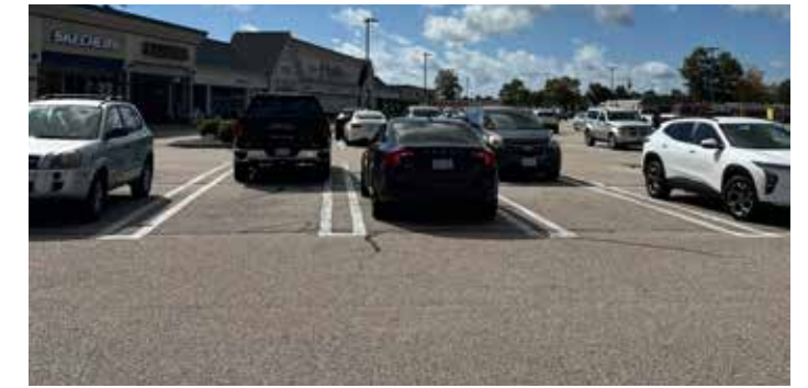
Excess impervious areas cause hotter temperatures and increased runoff. This parking lot could be retrofitted to add more trees, bioswales, and pervious surfaces that allow water to seep into the ground.
