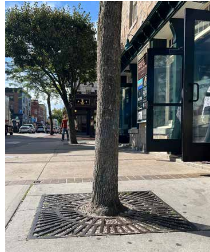
Small spaces for tree roots leads to unhealthy trees and less stormwater infiltration
