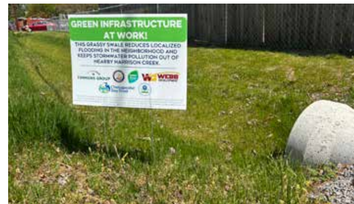
This grassed swale allows water to soak into the ground, thereby reducing neighborhood flooding and pollution of nearby Harrison Creek.
