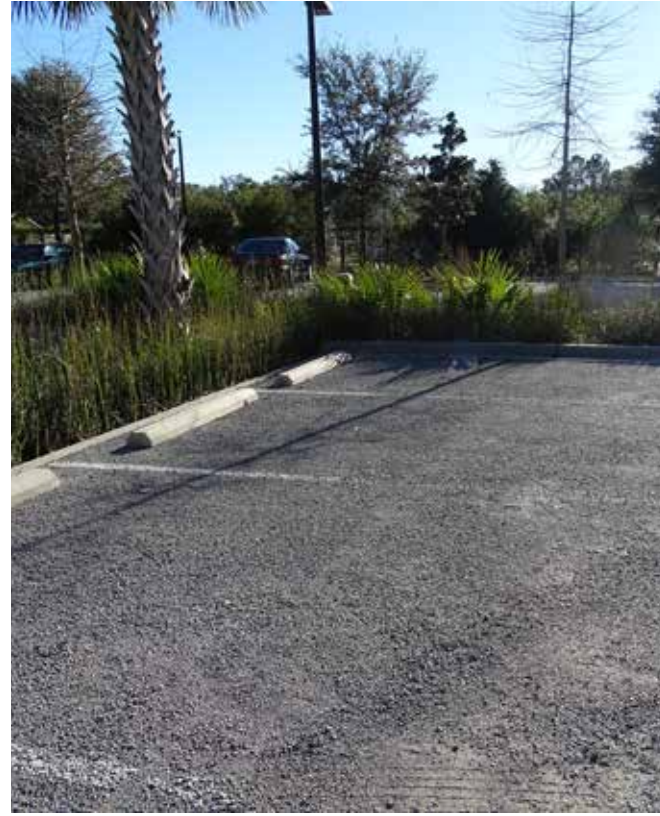
These parking lot “islands” in the City of Charleston are recessed and engineered as bioswales planted with trees to aid in filtering and evaporating stormwater. They also added permeable parking spaces too.
