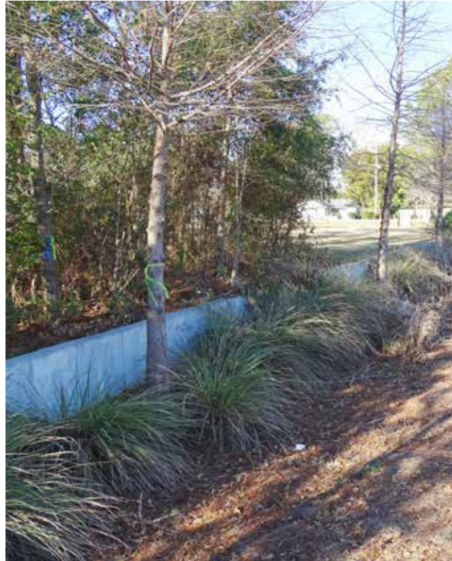
These parking lot “islands” in the City of Charleston are recessed and engineered as bioswales planted with trees to aid in filtering and evaporating stormwater. They also added permeable parking spaces too.
