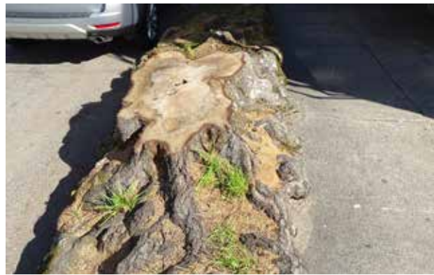
Urban trees suffer many challenges. This tree may have grown too large for its inadequate planting bed.
