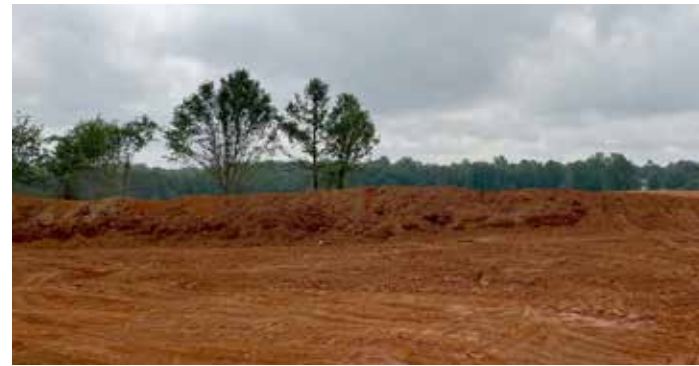
New developments are often cleared of most or all trees from a site before grading and construction begins. This results in a loss of a valuable resource that can support stormwater management, cleaner air and cooler communities.
